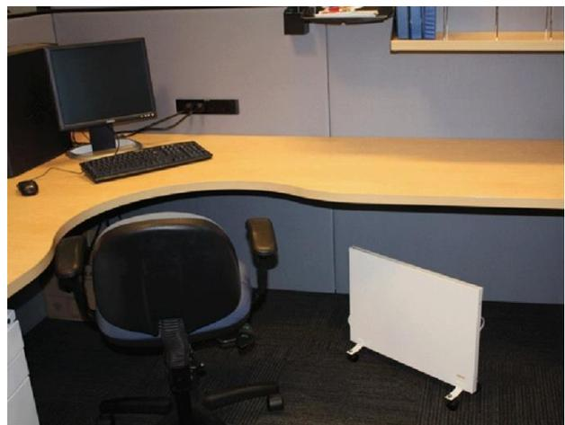
These heaters range in size. The model we use at UNSW is about 500mm long and 450mm in height. This is an ideal size to heat the legs of a person seated at a desk. A large proportion of the radiant heat produced by the unit will strike the person and be effective.
